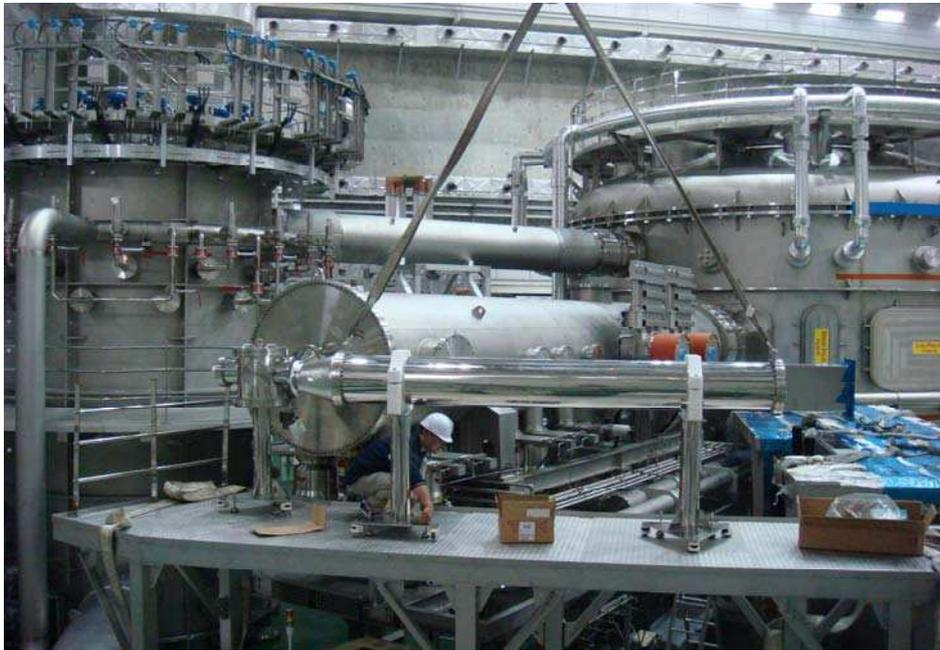
*Fig. 3. Installation activities for the fabricated XICS on the KSTAR tokamak.*
